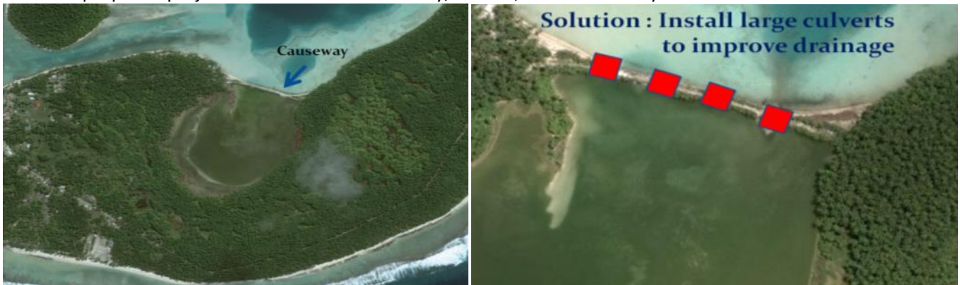
Causeway constructed across the Kuta cove of Rakahanga. This causeway is limiting the drainage of this Kuta watershed during flood events from both rain and high seas.
