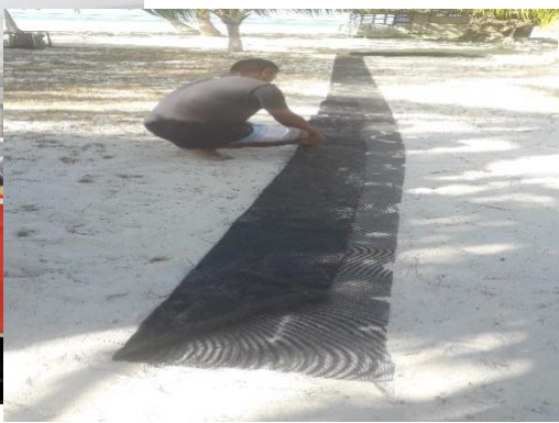
Figure 3: preparation for pen construction
