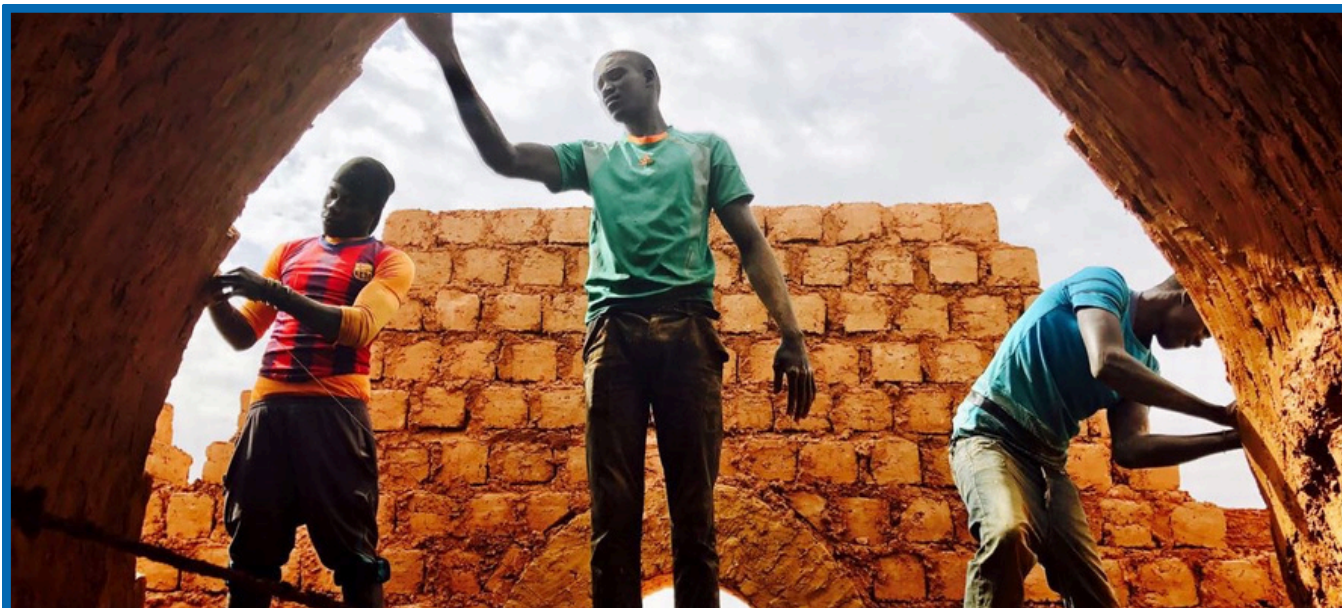
The Nubian vaults technique is highly climate adaptative and does not require any wood or timber - @AVN
