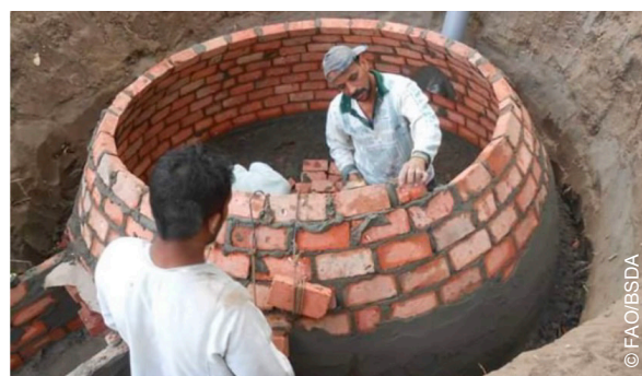
Figure 19. Anaerobic digesters to convert livestock manure into biogas in Behera (Nile Delta)
