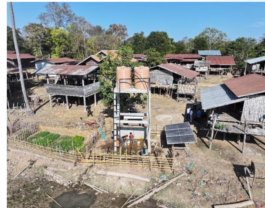
Groundwater well with Solar
