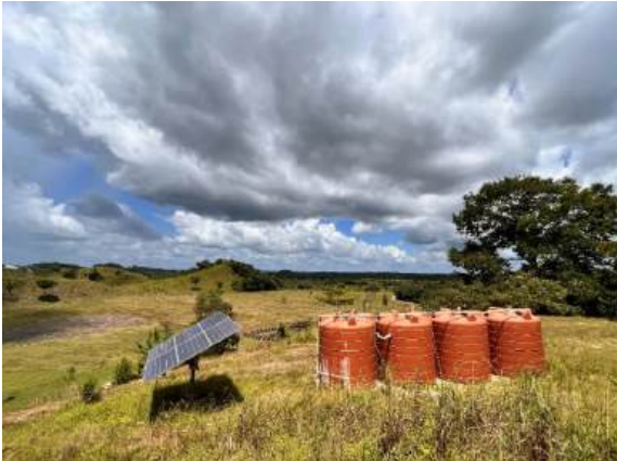
Figure 24. Breeder operation, solar power pump and tank in the Cayo District, Belize
