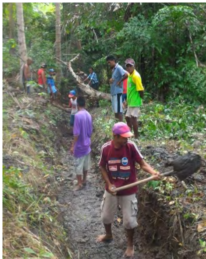
Figure 7 Villagers in Tarimbang Village, East Sumba are digging a new irrigation routes which will bring water closer to their villages
