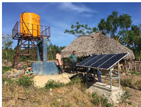
Figure 12 A Solar Powerd water pump in SPARC Village
