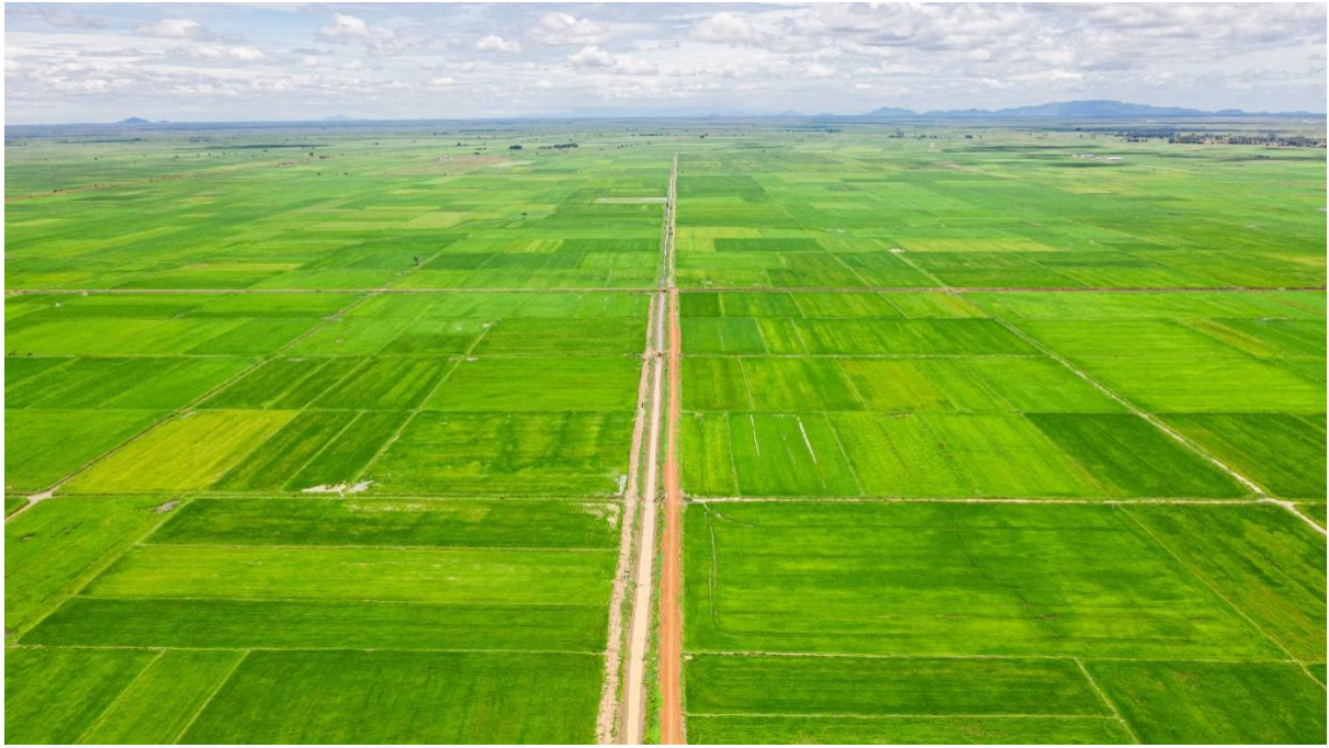
Aerial shot of rehabilitated canals in Thuol Jeat village.
