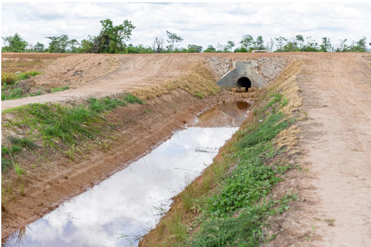
Newly rehabilitated canal in Laak village is ready to collect rainwater, but erratic weather patterns leave it sitting dry.
