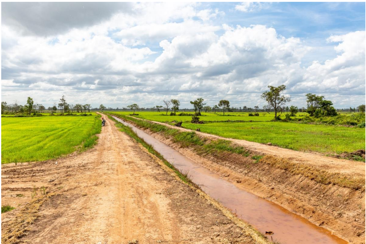
Canal rehabilitation projects have also led to the development of roads, helping to mobilise communities like Laak village in Santouk district.
