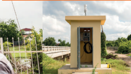
Automatic Weather Station and Automatic Hydro Stations in Kampong Speu Province
