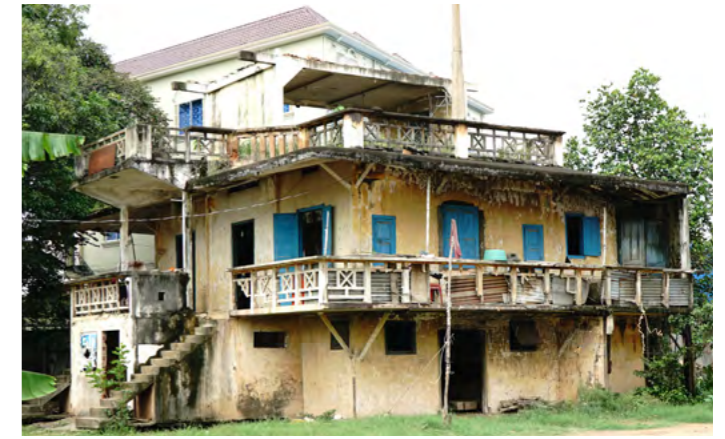
The old meteorology station building, legacy of the French colonial era.
