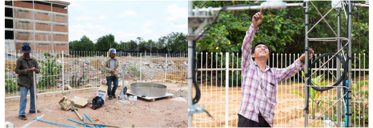
Installation of the station in Botum Sakor (left) and inspection of the equipment by Mr Nop (right)
