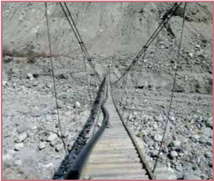
Pipe of Main Irrigation Channel Aliabad Hunza
