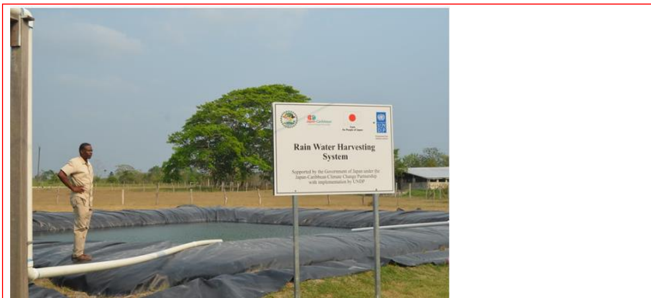
Belize – B1-Climate Smart – Finalisation of Water retention pond 14X14X3 meters at Yo Creek. This system provides additional water storage capacity of 400,000 litres/105,668 gallons
