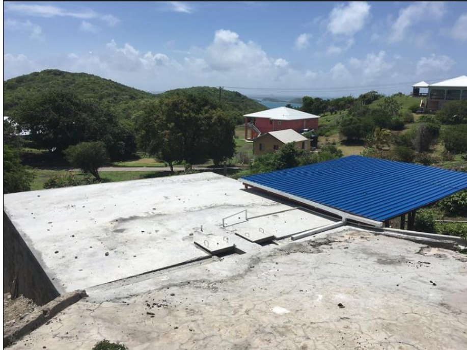
St. Vincent: SV1-Mayreau – Rehabilitation of cistern at Mayreau Primary School
