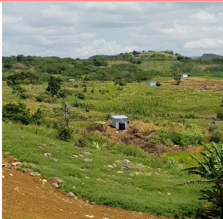
Jamaica: JM3-Cascade/St. Ann – Aerial view of 4 of the 50 tanks and sheds installed at this project. These tanks are allowing 50 farmers an additional 50,000 gallons of water storage for use in the increasing dryer times for agricultural production
