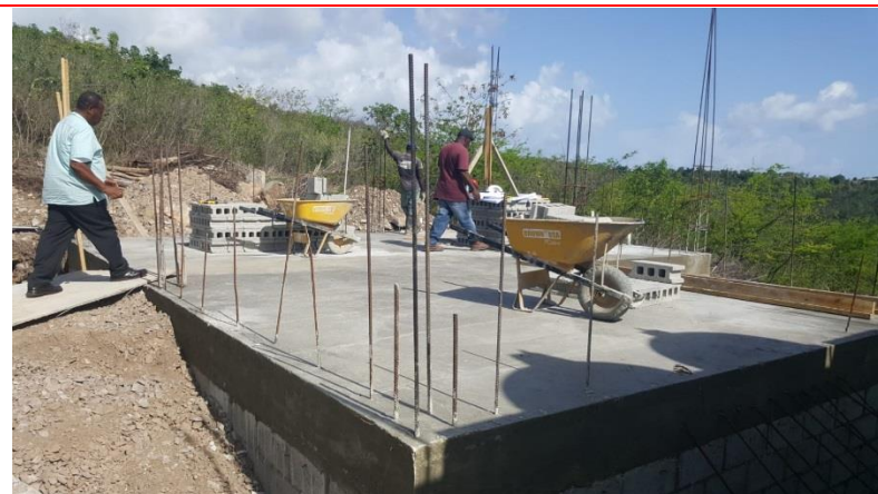
Dominica: D4-Morne Rchette – Construction of Emergency Operations Center. Blockwork for walls about to commence. Construction end date scheduled for August 31 st 2019.
