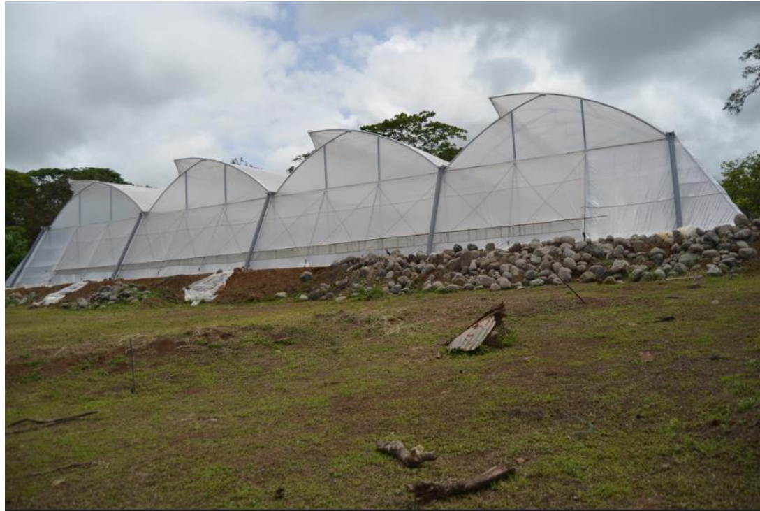
Grenada: GN5-Mirabeau. 95 x 121 ft Greenhouse installed at the propagation station
