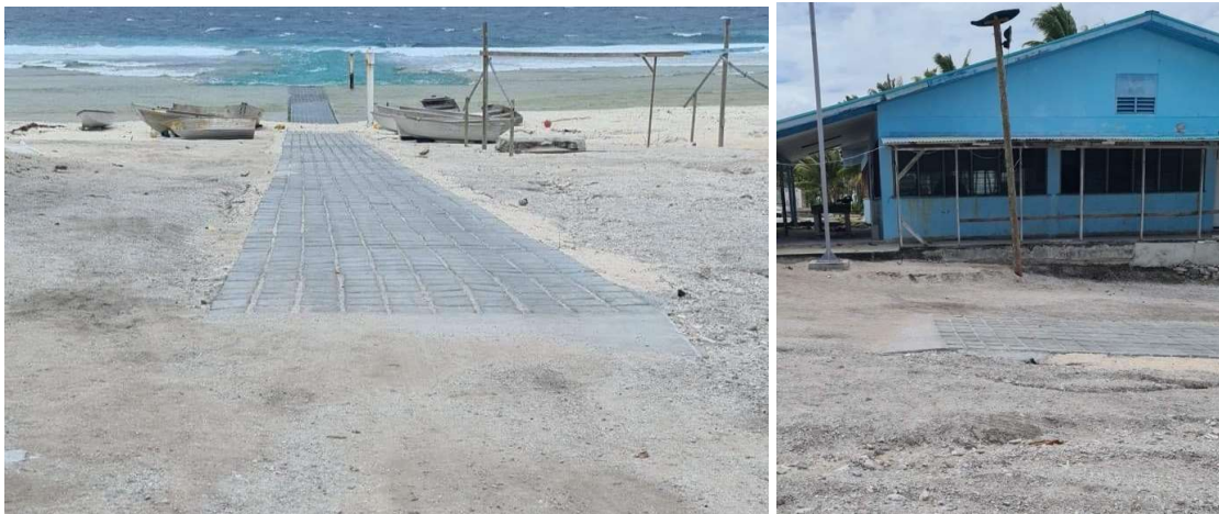
Figure 10: recently constructed Flexmat™ cellular concrete boat ramp on Nanumaga.
