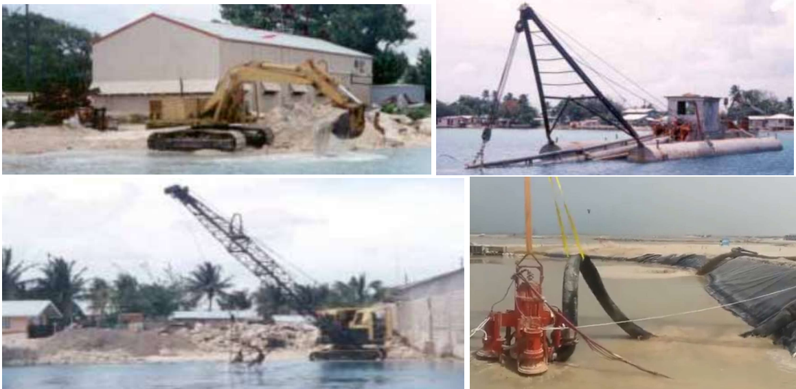
Figure 13: Examples of sand extraction methods from atoll lagoon environments. Clockwise from top left: shore-based hydraulic excavator, pontoon cutter section dredge, submersible drag flow pump with cutter-suction head, drag line operated from shore-based crane. (Image sources: Smith (1995), www.sandredger.com )
