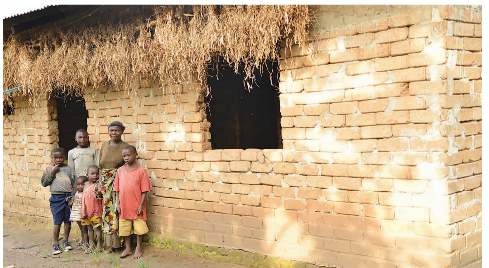
Joanita Gumonye with some of her children stand in front of their new house built with the unbaked bricks. On the right side is their old house (Photo: UNDP Uganda 2014).
