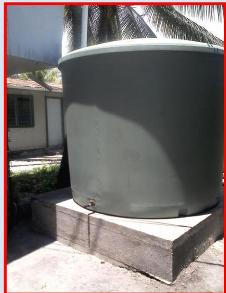
**Photo (above):** These tanks are now popping up within the community on the isolated Palmerston Pa Enuu. The concrete tank bases are something that was not done in some of the other past water tank projects. Lessons have taught us of overflowing water scouring away sand bases causing tanks to tilt and tear.
