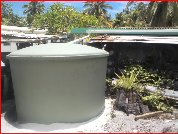
**Photo (above):** This installation on Palmerston Pa Enea was an acceptance. The roof to the catchment area was approximately 1.400 meters high; the tank had to be buried approximately 1.000 meter in the ground with a channel dug out for the tank owner to collect water through a tap in the tank base. The tank been buried in the ground also minimised the chances of tilting.
