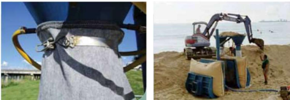
Figure 46: Details of 2.5m<sup>3</sup> GSC units, schematic and images of GSC coastal structures during construction (source: Elcorock , 2019 and AECOM)
