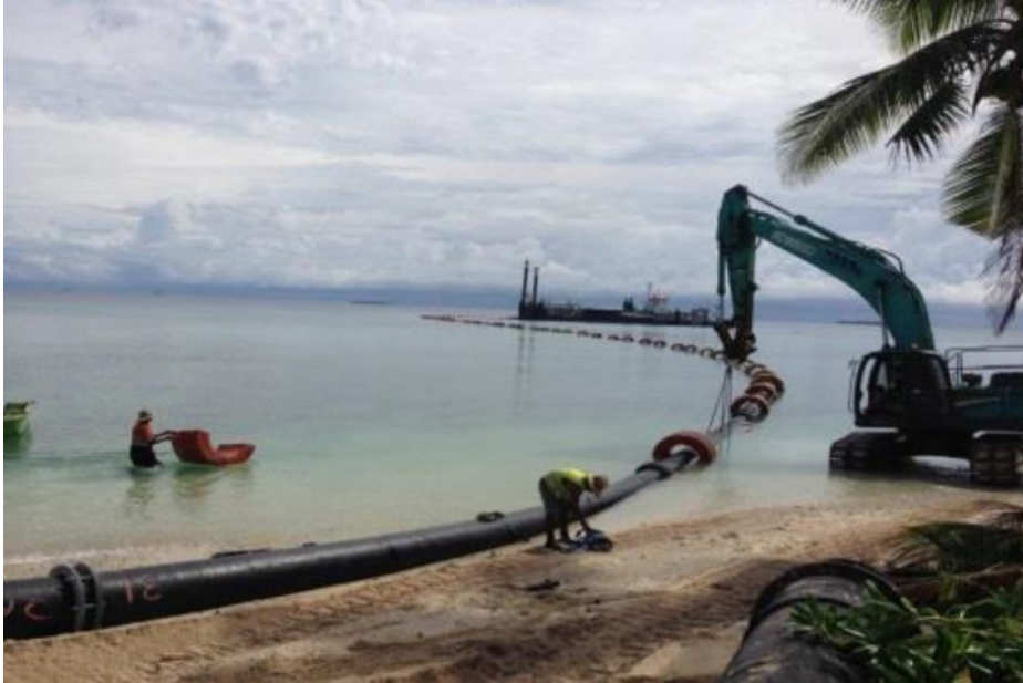
Figure 12: Dredge pipeline on shore for the Tuvalu Borrow Pit Reclamation Project. Source: Hall Contracting
