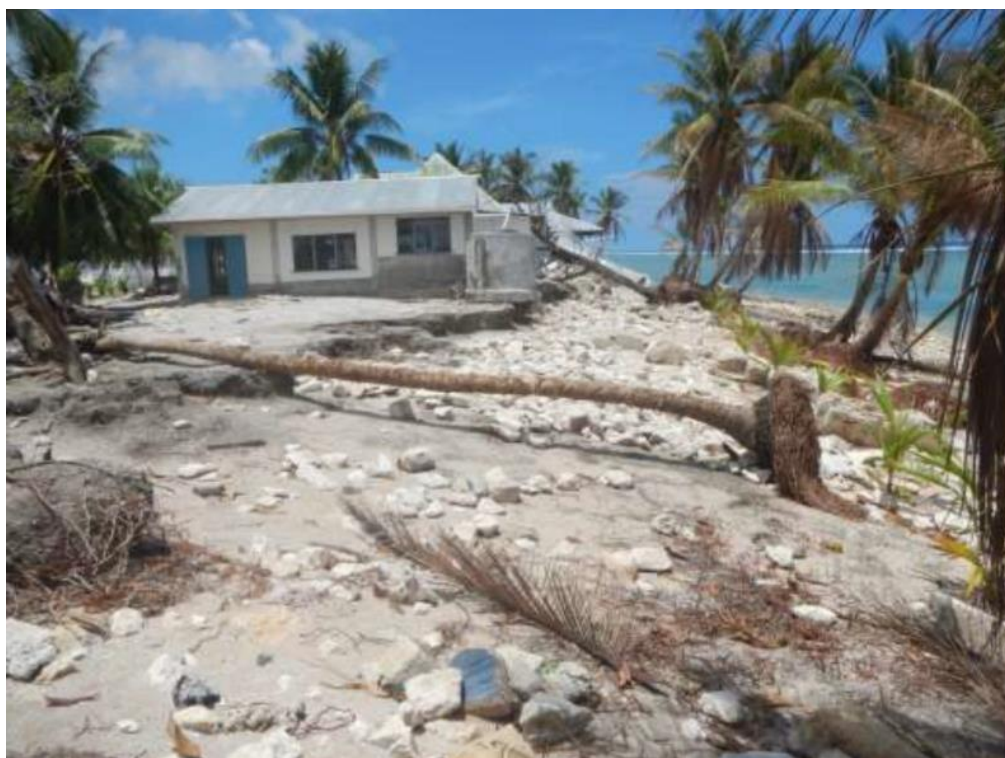
Figure 33: House undermined and eroded on Nanumea
