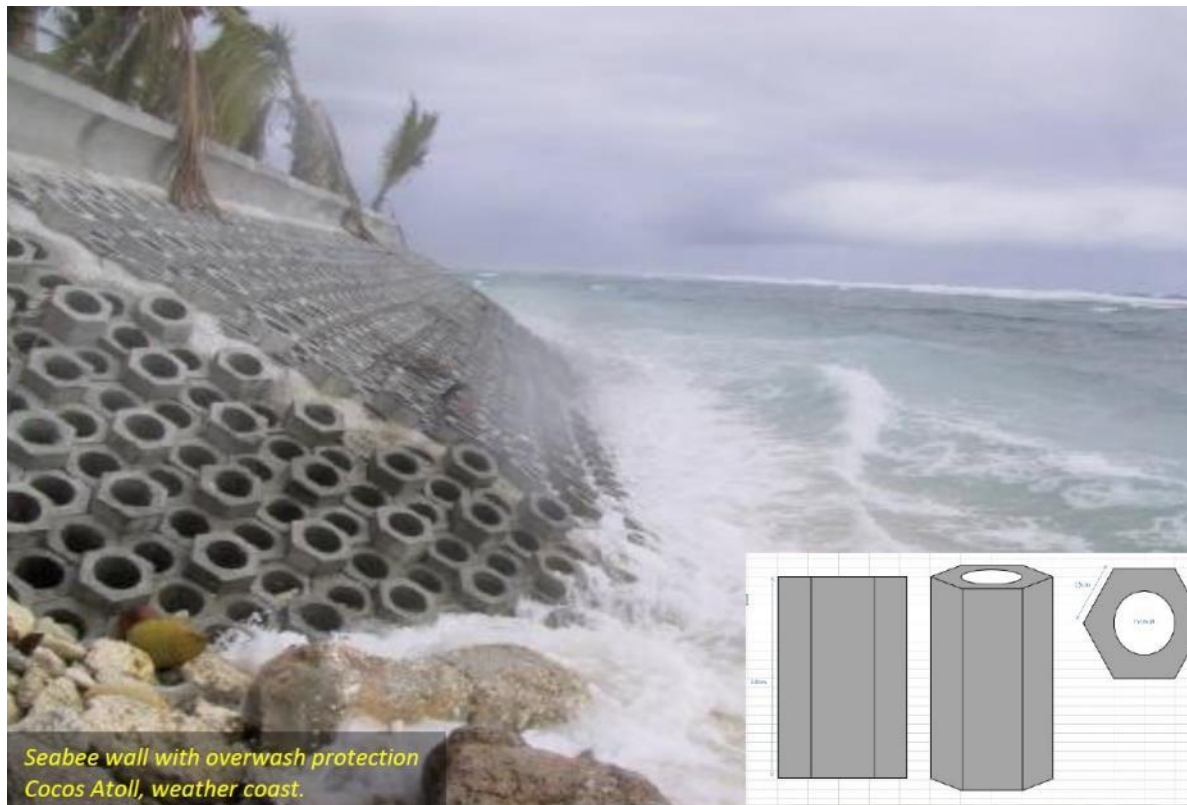
Figure 14: Seabee wall installed in an example location
