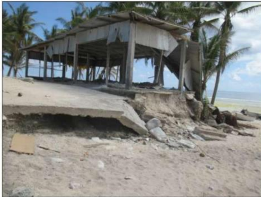
Figure 32: Erosion on the western foreshore of Nanumaga following TC Pam
