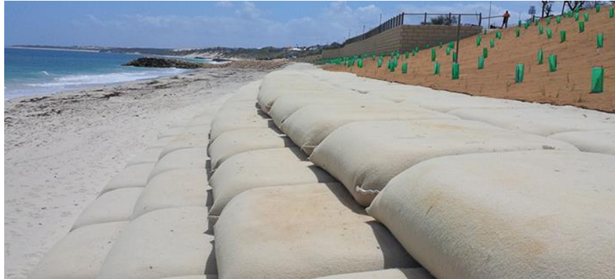
Figure 17: Example of back of beach geo-textile revetments
