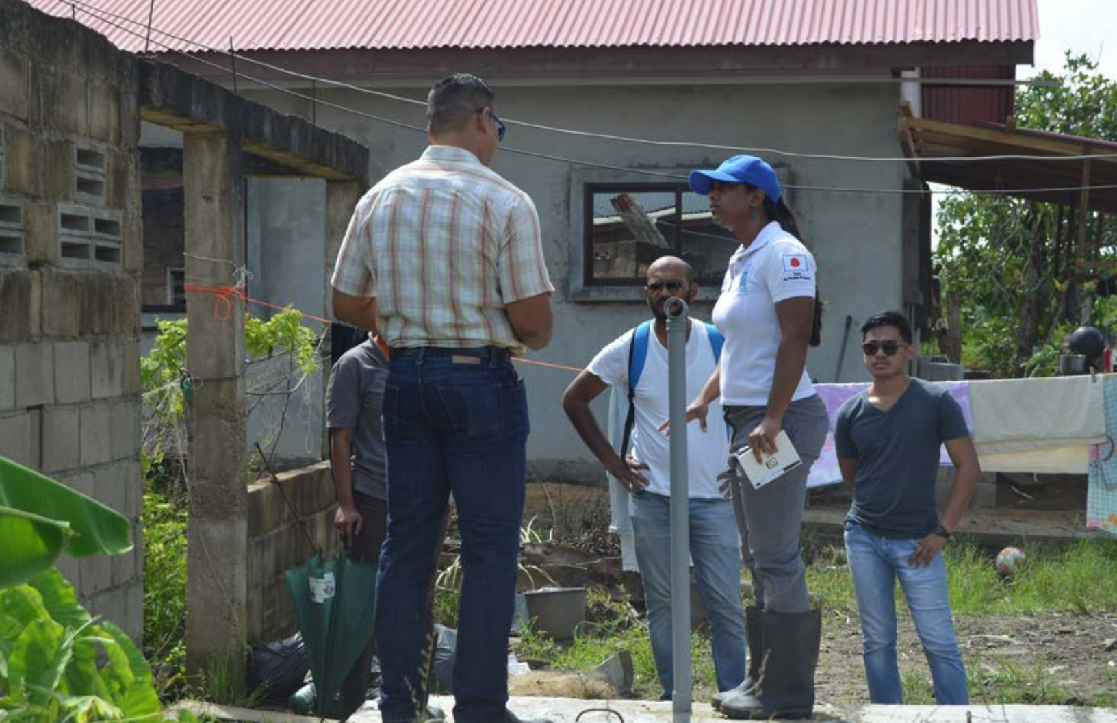
The project team stands on a newly installed septic system, while discussing the project's progress
